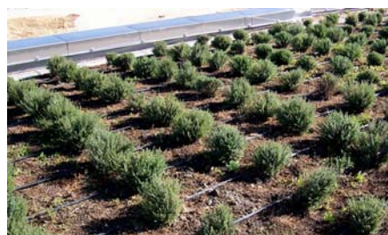
A drip irrigation was installed on all roof surfaces.
