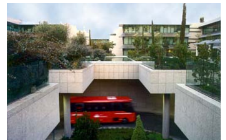
Driveways for cars and buses under the green roof area.
