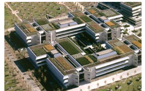
The aerial view shows the different planting areas with their own character.
